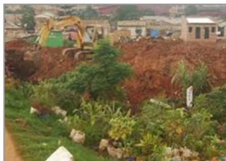
Constructing houses in wetlands.
